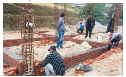
that will form the main structure of the building. Once this is complete, we will begin the brickwork phase forming the exterior walls of the classroom block.
