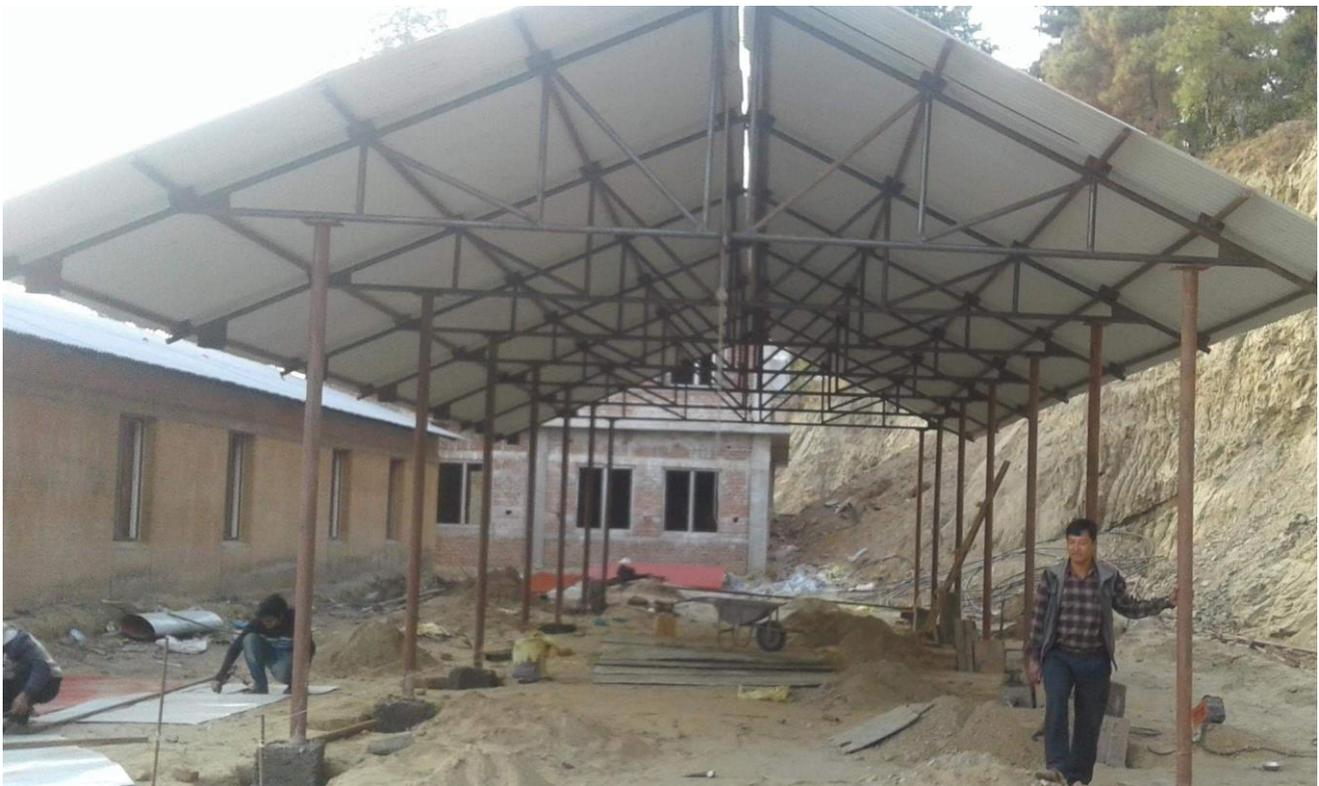
Before the monsoon, we delivered 8-9 truckloads of materials which included the entire metal framework, corrugated metal roof panels, high quality timbers for windows and doors, cement, rebar, and local materials like sand and aggregate.
