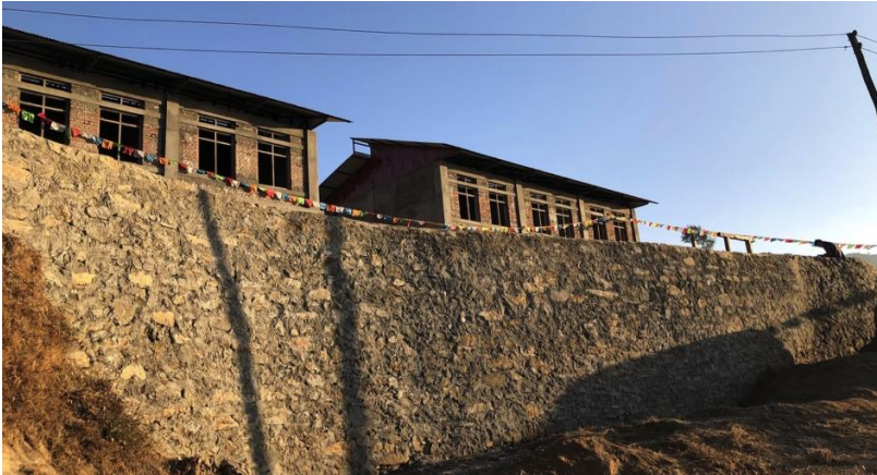
Figure 6: The completed wall which was constructed to retain land vulnerable to landslides
