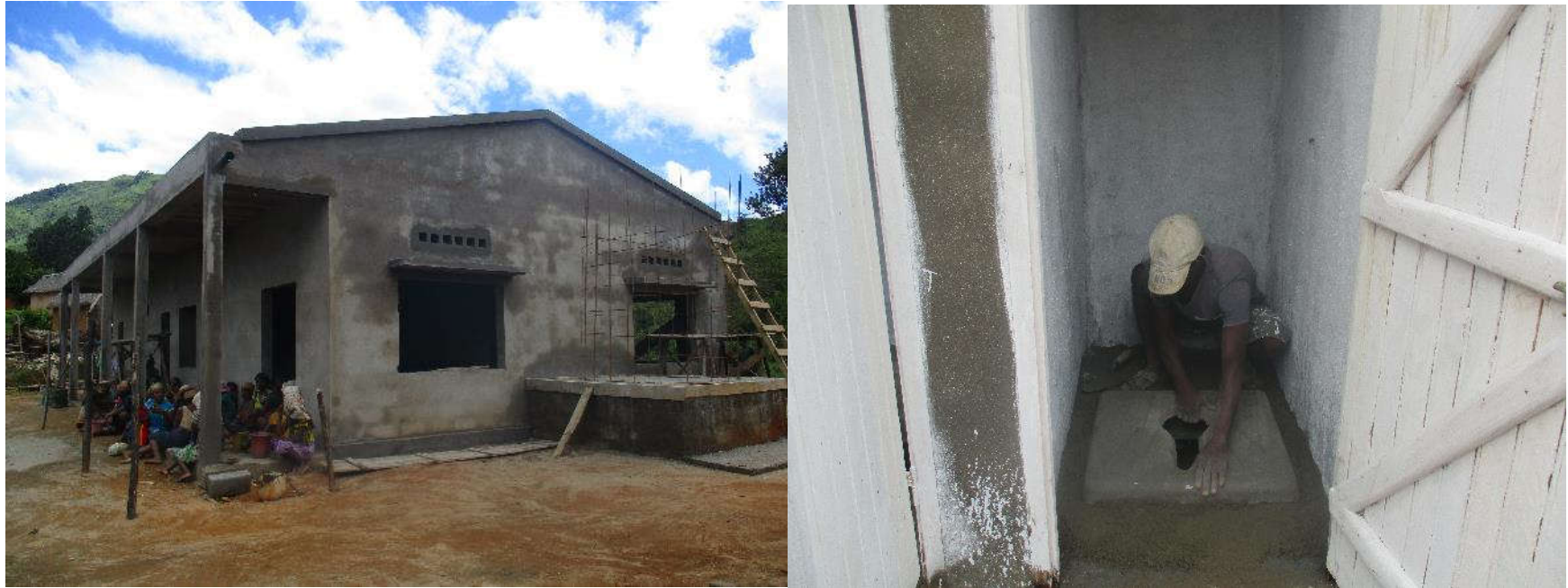
Progress with building work in February 2019
