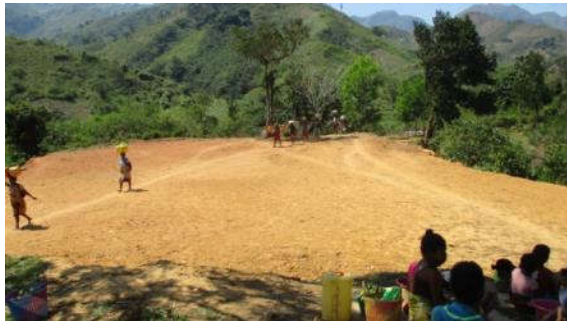
The building site already levelled and ready for building.
