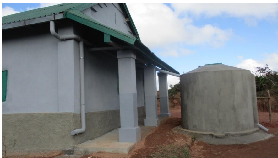
The renovated impluvium rainwater catchment system
