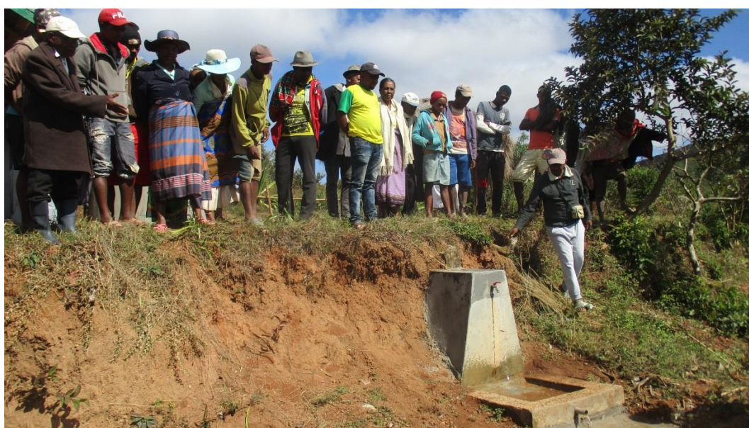
The newly-renovated and functional tap-stand, linked to the rainwater catchment system.
