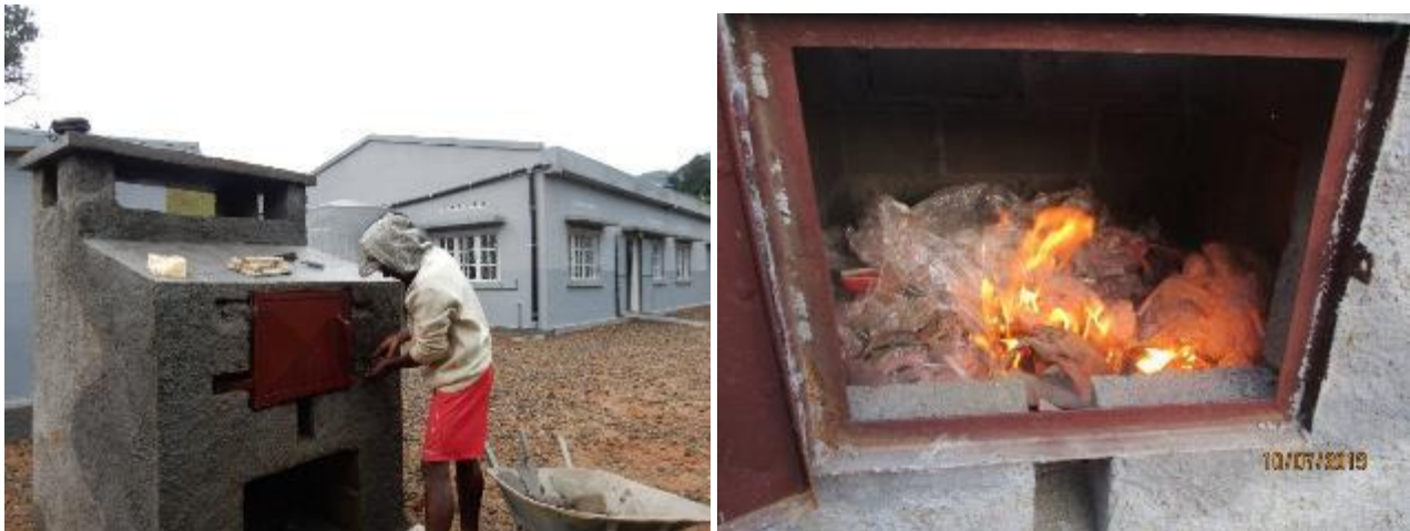
Figure 33: Finishing touches to the incinerator (left) & it in use (right).
