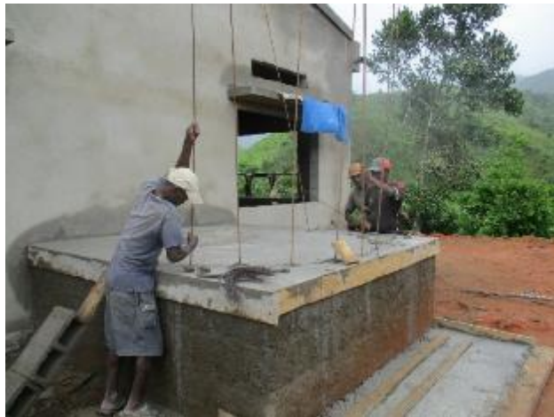
Making the ferrocement impluvium rainwater catchment tank:
