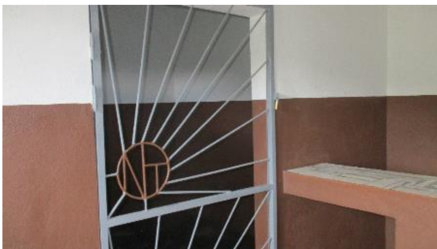
Figure 23: Protective door grid to the storeroom.
