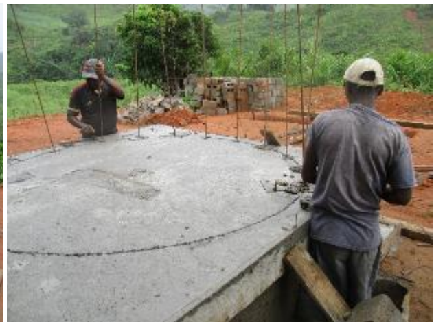
Making the ferrocement impluvium rainwater catchment tank:
