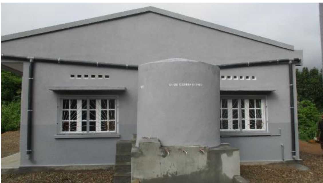
Figure 24: The rainwater catchment system at Mamolifoly Health Centre.
