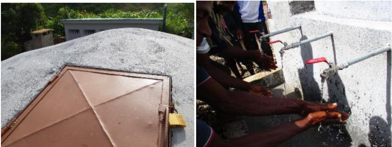
Figure 27: The hand-washing points linked to the impluvium rainwater catchment system.
