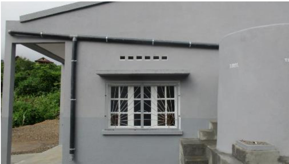
Figure 24: The rainwater catchment system at Mamolifoly Health Centre.
