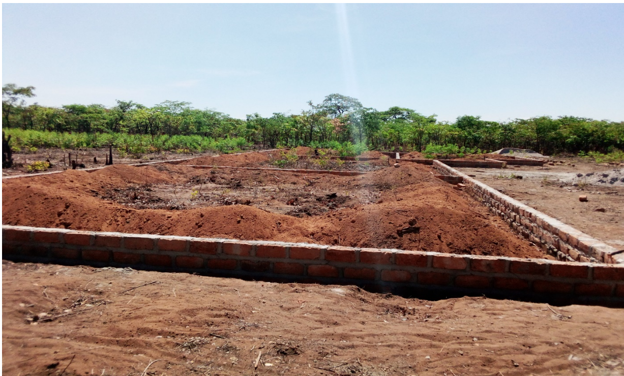
This is the box waiting to be filled with gravel
