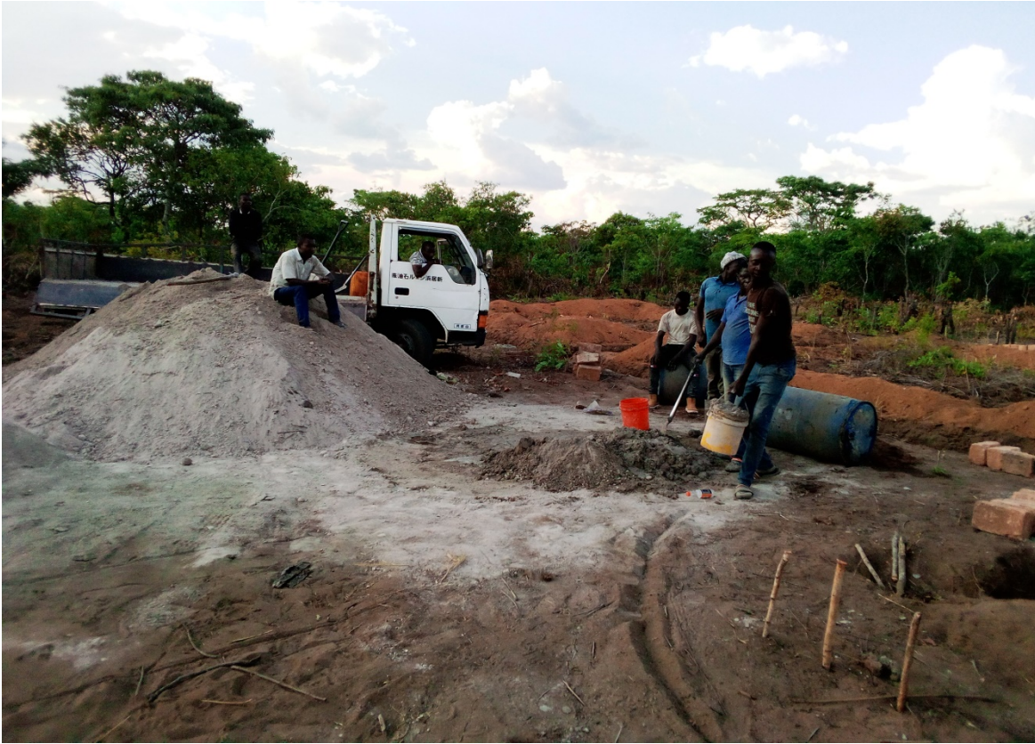
The transporter ferrying sand and helpers mixing mortar
