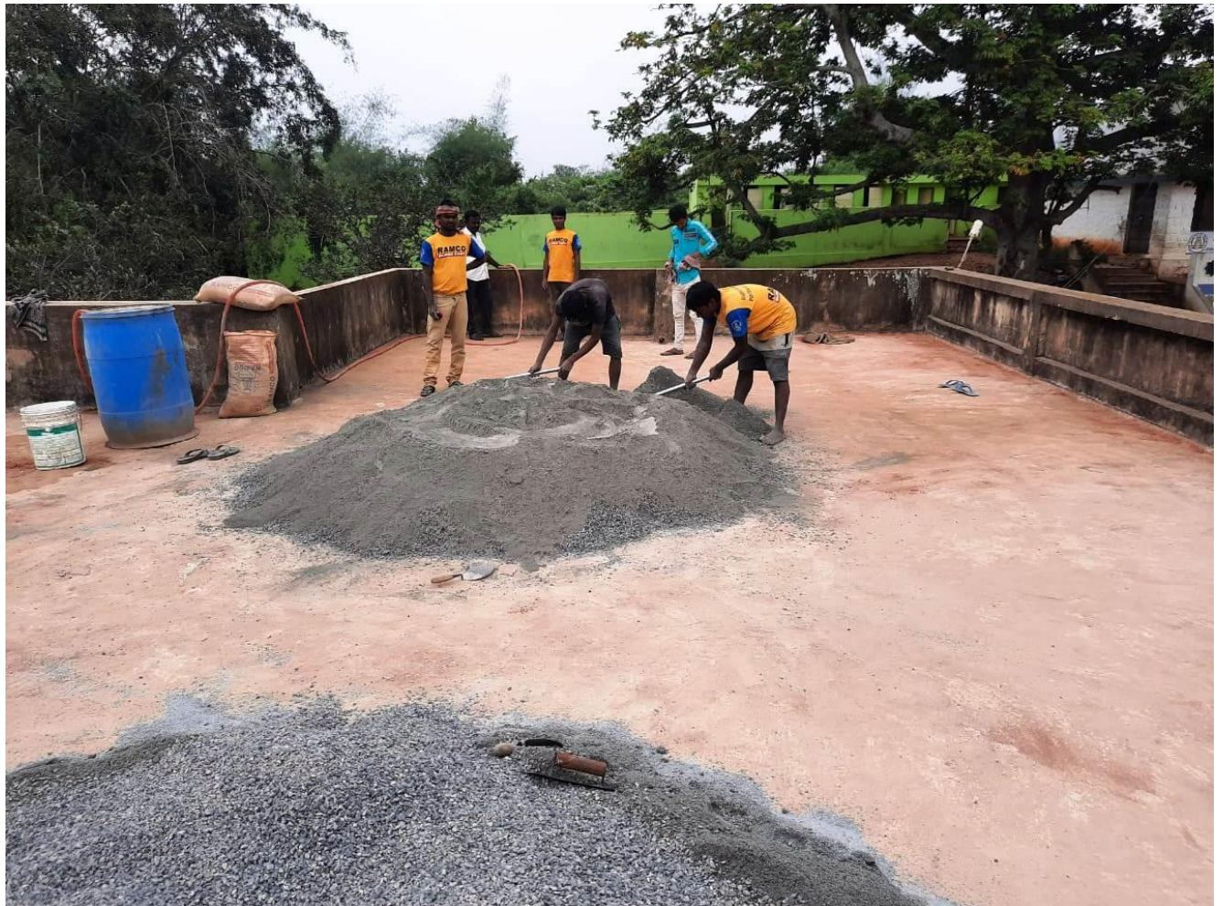
The process of laying the weathering course with R.C.Concrete mixer
