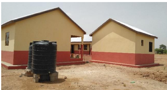
Completed Cheshugu primary school showing water tanks and aprons.
