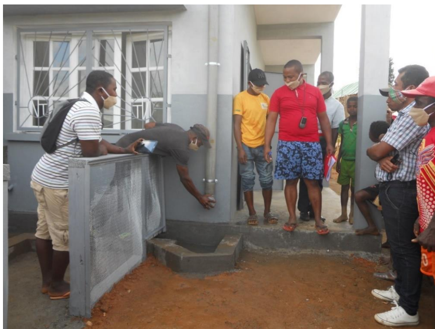
Figure 23: The down-pipe 'disaffection' system to prevent the first rains (which bring dirt from the roof) from entering the water tank.
