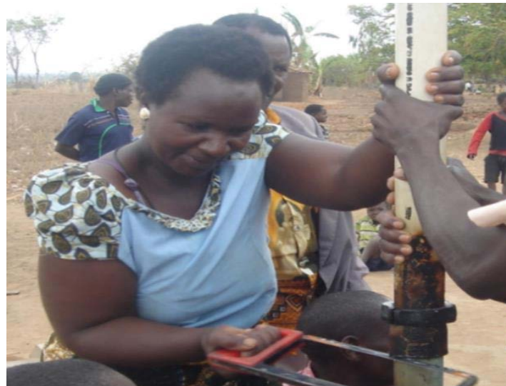
Olepolos Pump. Picture showing a woman being trained as the cylinder was pulled out for repair.
