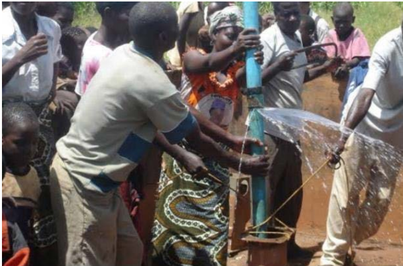
Osenai Pump. Pulling out of risers to repair a leaking pipe.
