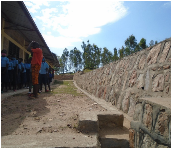
Fig. 1: The retaining wall
