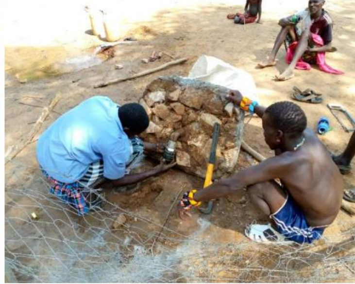
Building a more robust concrete plinth
