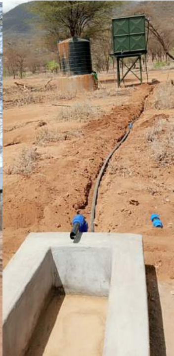
New pipeline to trough
