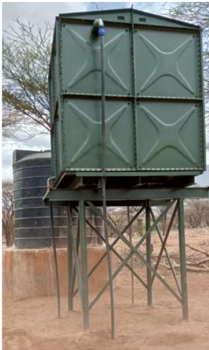
The new steel tank
