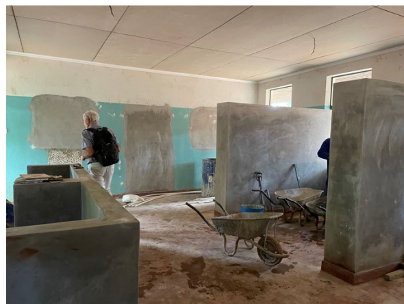
Construction & plastering of individual patient bays.
