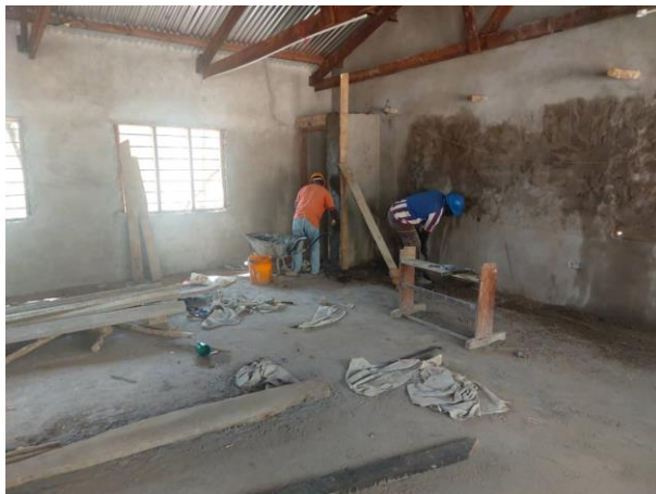
Internal Plastering
