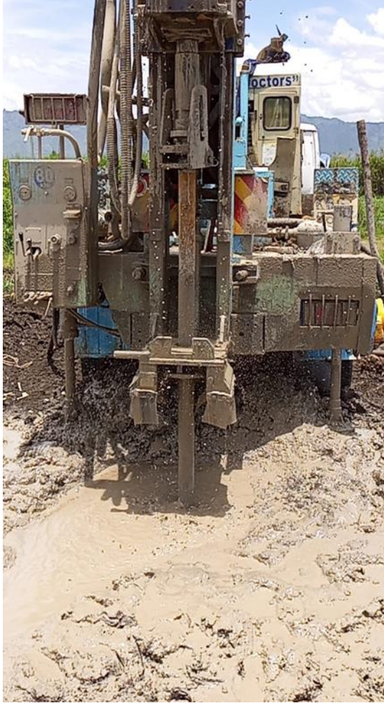
Mud drilling process at Yago Primary
