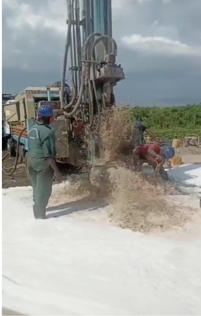
Flushing the well with the rods to remove the cuttings
