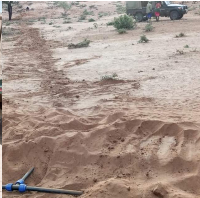
Supporting the pipeline installation
