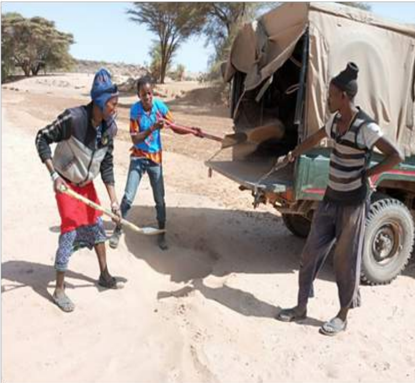
The vehicle collecting sand for concrete
