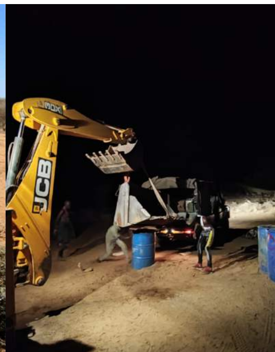
Unloading the newly repaired bucket
