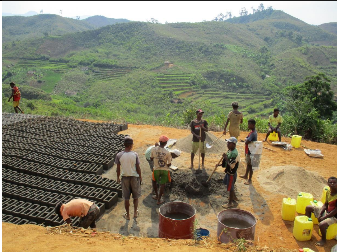
Making the cement breezeblocks in Maromby.
