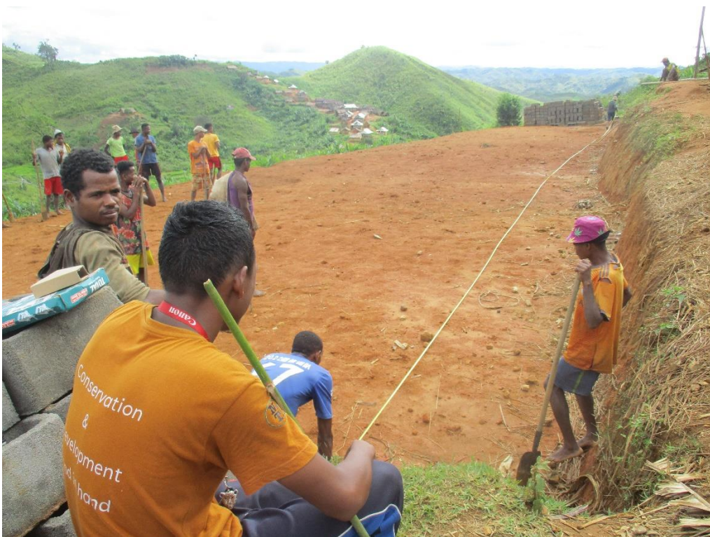
Situation after initial levelling-of-land (above) and (below) marking-out additional levelling-of-land required.
