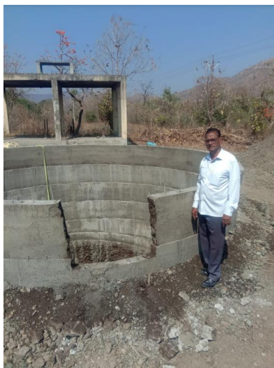
Construction work of the open well in Vetawadi
