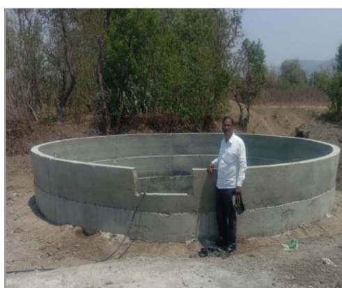
Completed construction work of the open well in Rampurwadi
