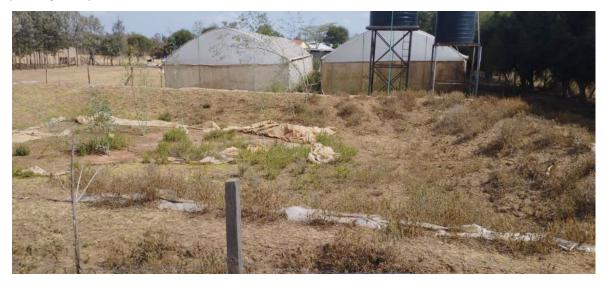
The pre-construction phase involved digging out the worn out dam liners, vegetation, and all the materials deposited into the ponds. This was intense manual work and it took a week to clear the 2 reservoirs.
