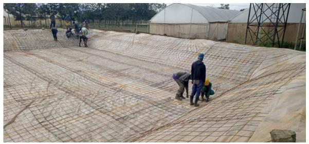
After the curing of the base, timber formwork was fixed to allow concrete to be poured to form the sloped sides of the reservoirs.
